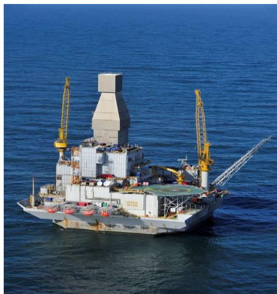
The Orlan power generating system is designed to provide power supply for all electrical equipment including those supporting production processes, engineering systems, drilling operations and living quarters. The system configuration was designed with consideration for various operating modes, such as normal and emergency operations and cold start-up. The platform has power generation system of two types:
