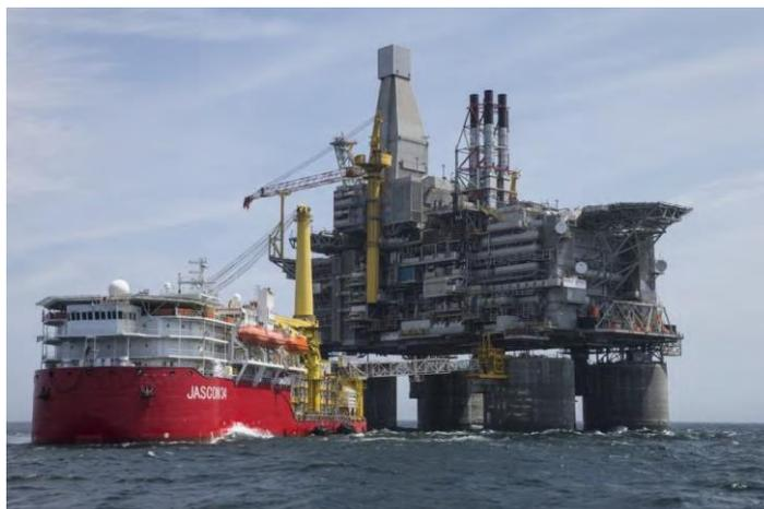
The platform consists of a gravity base structure holding a derrick, steel structures with production equipment, living quarters, cranes and a helideck. Berkut was installed in June 2014 and started production in 2015.
