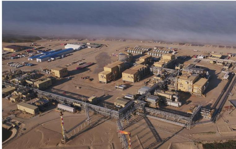
Odoptu has an independent power supply system with the gas turbine power plant used as the main source of electrical power. The facility also has three diesel power plants of equal capacity. They are the independent source of power supply and are constantly ready to start up and take over the load. They are intended for emergency power supply.
